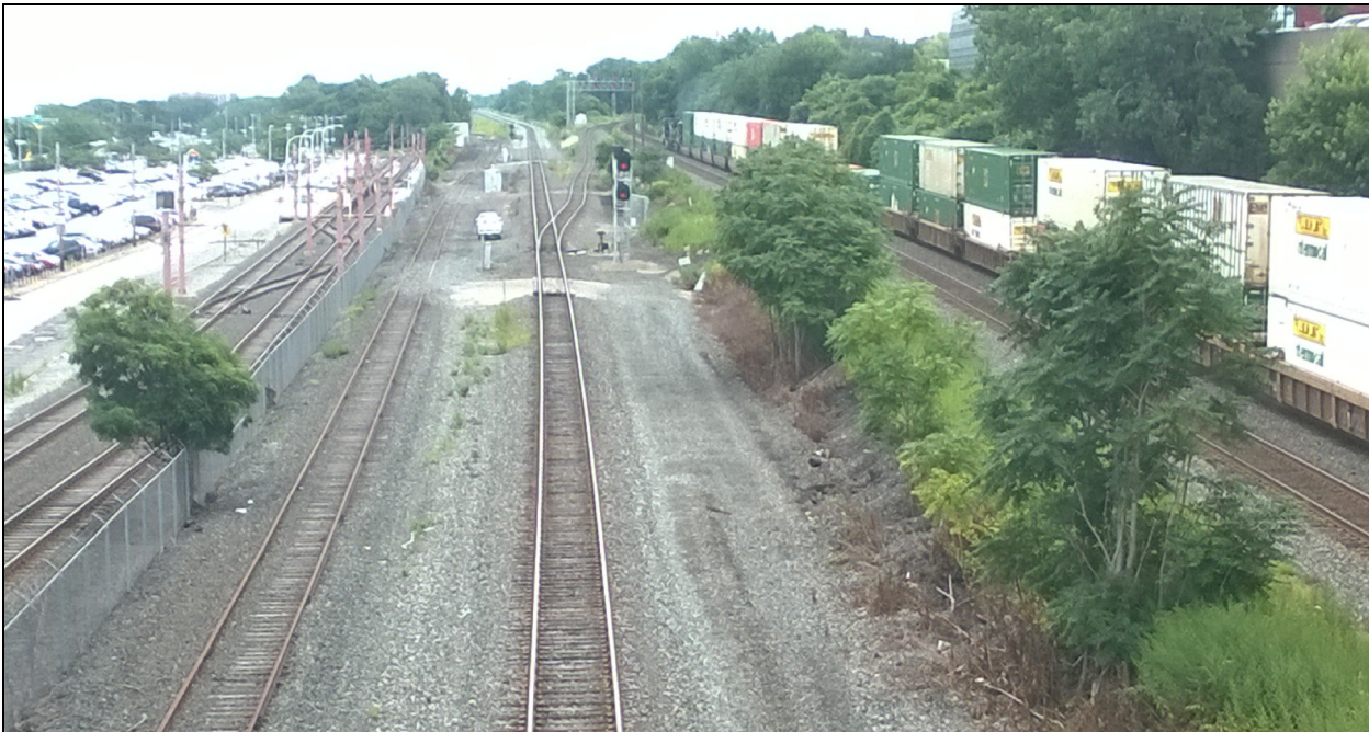
Looking east from the North Point Building's pedestrian walkway, the tracks from left are GCRTA's two-track Waterfront Line, CSX's Track 44 (owned by NS west of here), NS's Amtrak Connection that climbs the gradient past CP181's double-red signal (CSX's Cleveland Terminal Subdivision continues straight ahead) to CP122's signal bridge, and NS's Cleveland Line Track 2 and Track 1 (the latter being used by the double-stack intermodal freight train).
