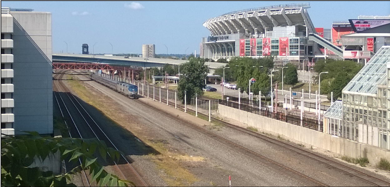
Looking west from East 9 th Street toward Cleveland Browns Stadium, Amtrak station and, at far right, the Greater Cleveland Regional Transit Authority's (GCRTA) North Coast station. Tracks from left are Norfolk Southern's NS Cleveland Line Track 1 and 2, NS's Amtrak Connection track (on which the Amtrak train is setting next to the station platform), Track 44 (owned by NS west of East 9 th and CSX east of East 9 th ), and the GCRTA Waterfront Line tracks (not visible).
