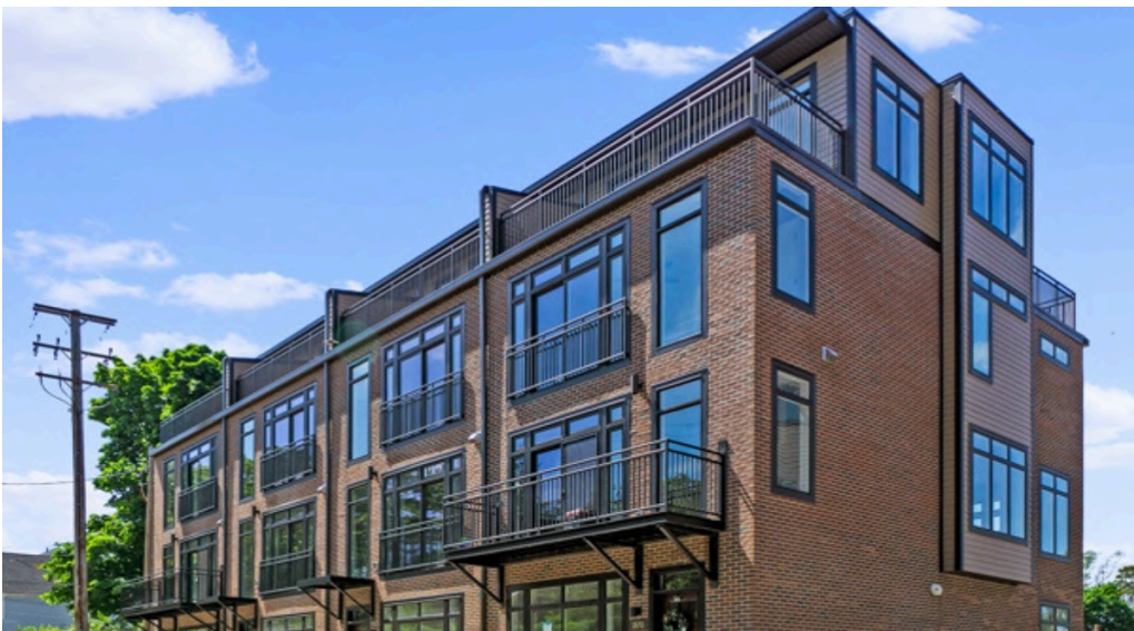
Woodhill Townhomes - E120th & E123rd Streets -Contemporary Example: Fourth Story is setback, providing a generous balcony.
